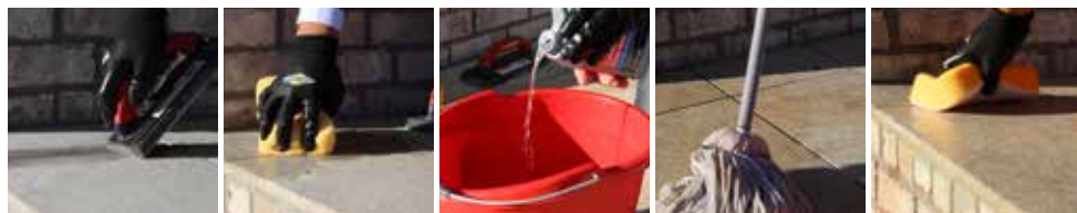
PIC 1. Fill joint with grout.
